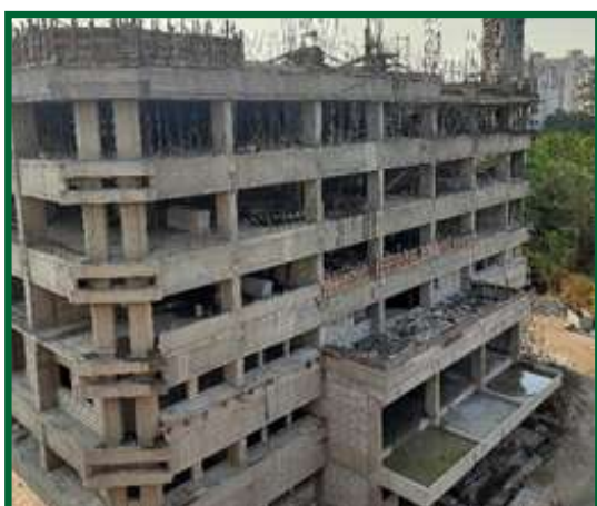
Construction in progress for Niyamak Bhavan-C at Mumbai
